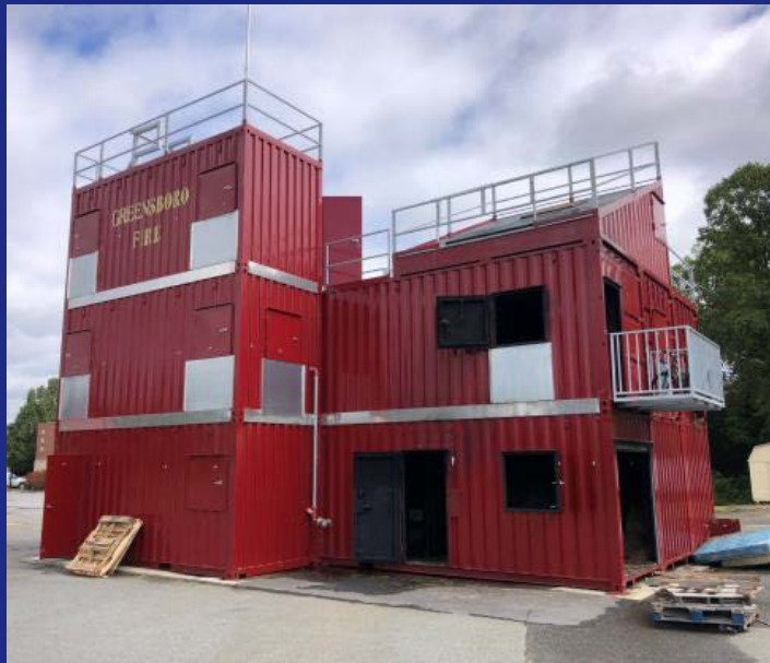
Fire training tower/Burn Building
