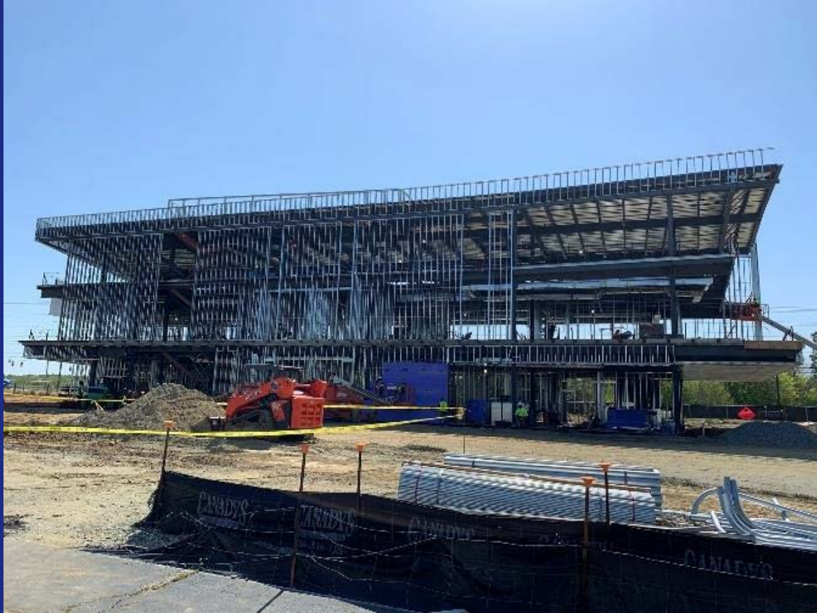
West side of building
